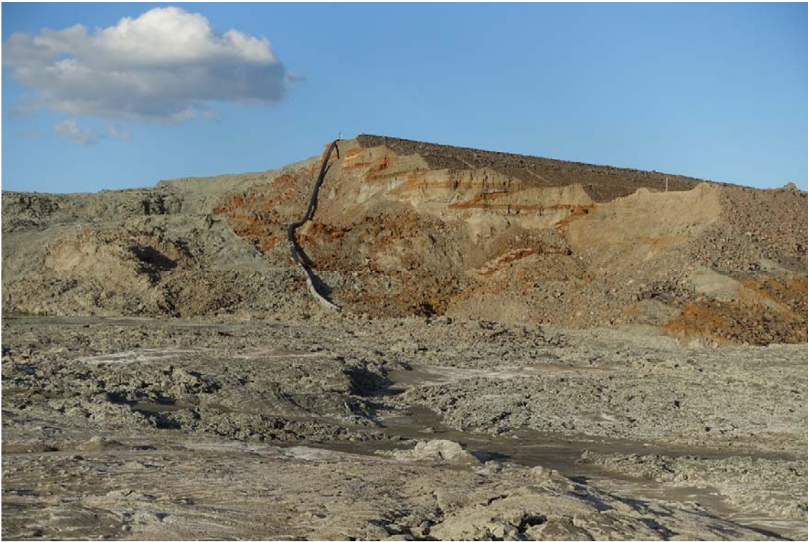
Photo B8-8: Left abutment showing well-constructed and clear embankment zoning.
