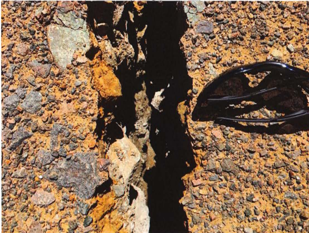
Stage 8 crest, close-up of crack opening (IMG_2526)
