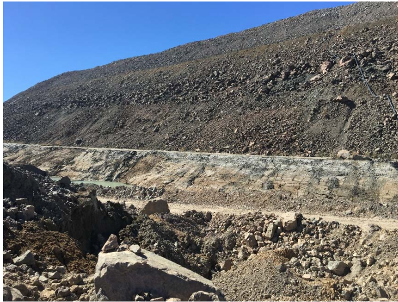
Photo B8-5: Cracking of excavated face in tailings at Chainage 2000 (2018-009)
