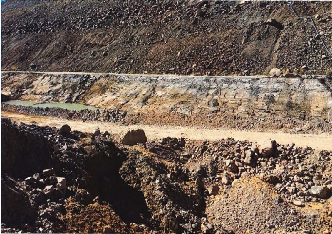
Toe area, linear cracking on exposed batter, looking westwards (IMG_2538)
