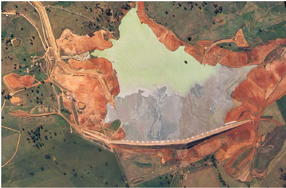
Photo B2-1: Stage 1 NTSF extents showing stripping (1998 Aerial Photograph) (1998-002)
