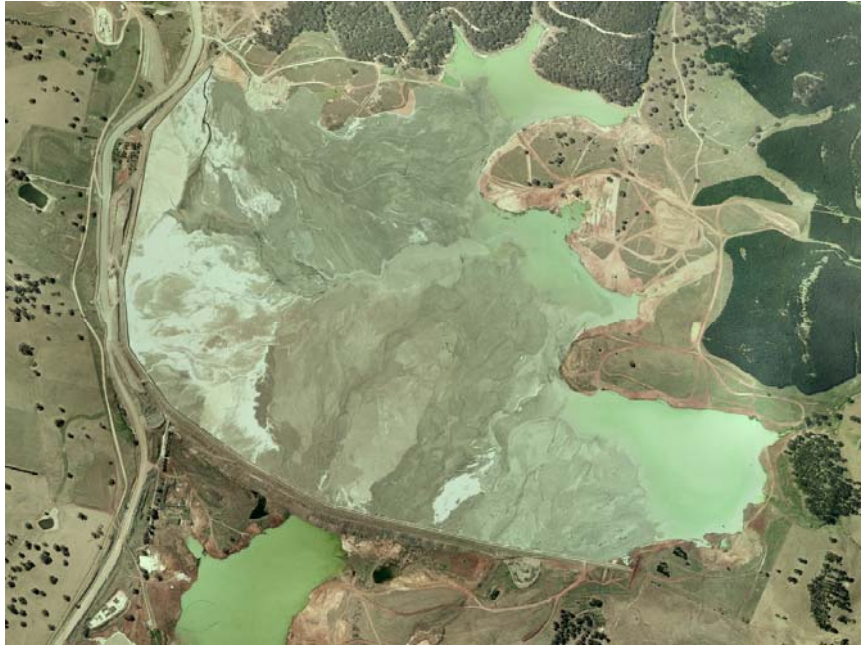
Photo B2-2: 2006 Aerial photography showing Stage 3 arrangement (2006-002)
