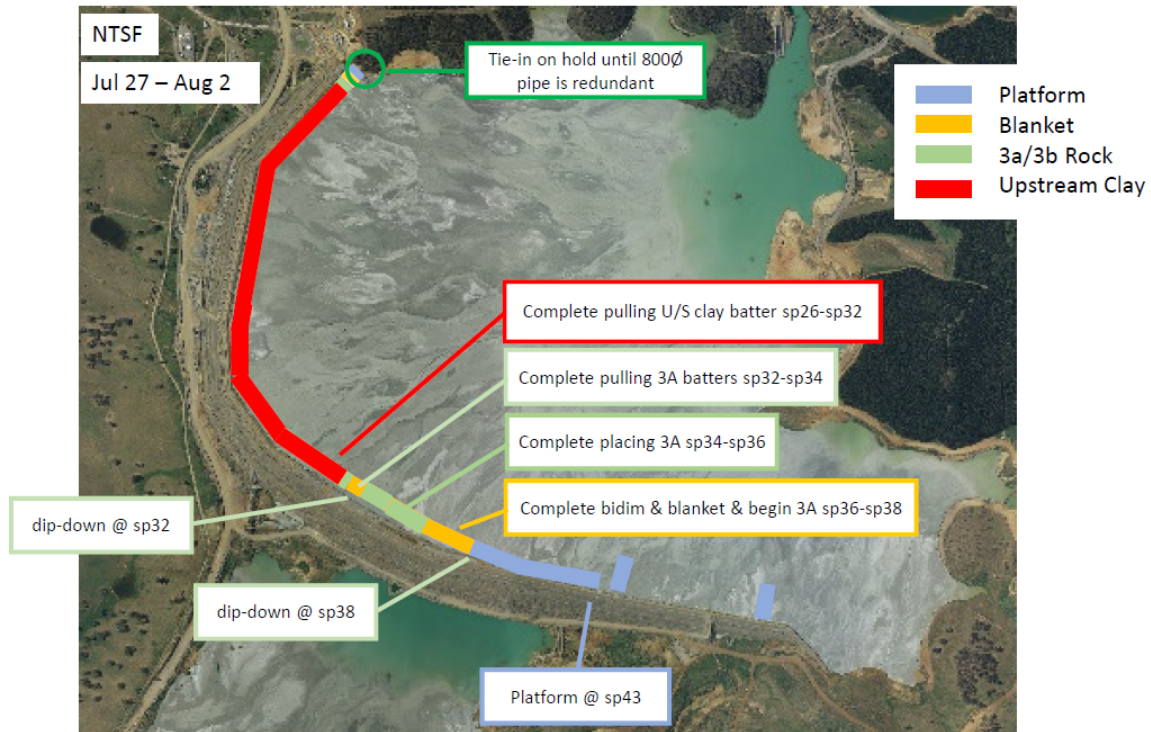
Photo B2-4: Proposed Stage 10 Construction WE 02 August 2017 (2017-008)
