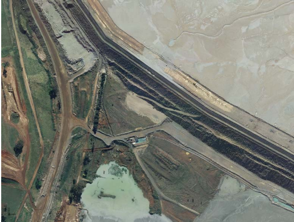
Photo B2-3: Downstream of NTSF embankment (2010) (2010-001)
