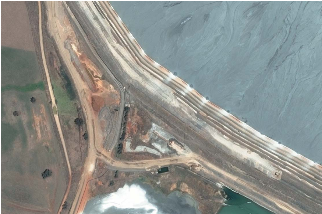
Photo B2-5: Stage 1 Buttress construction on 18 January 2018 (2018-002)
