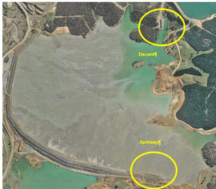
Figure B7-1: NTSF showing spillway and decant pond
