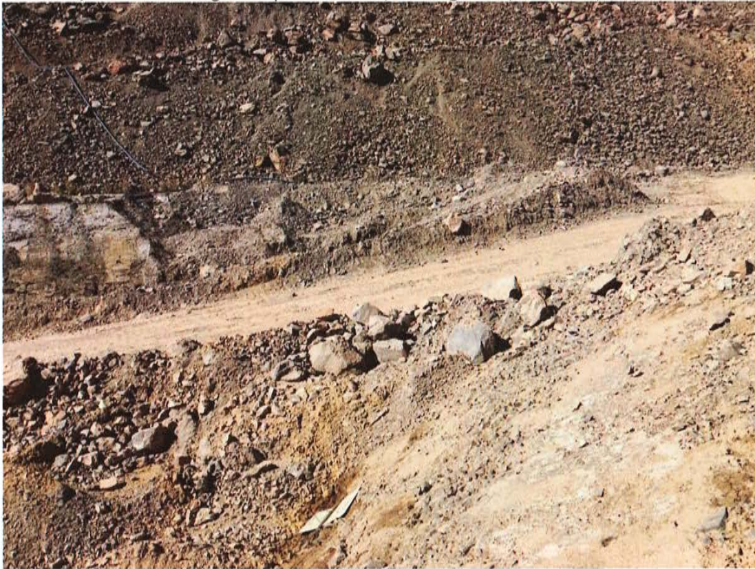
Toe area, linear cracking on access road (ground rupture), looking NE (IMG_2540)
