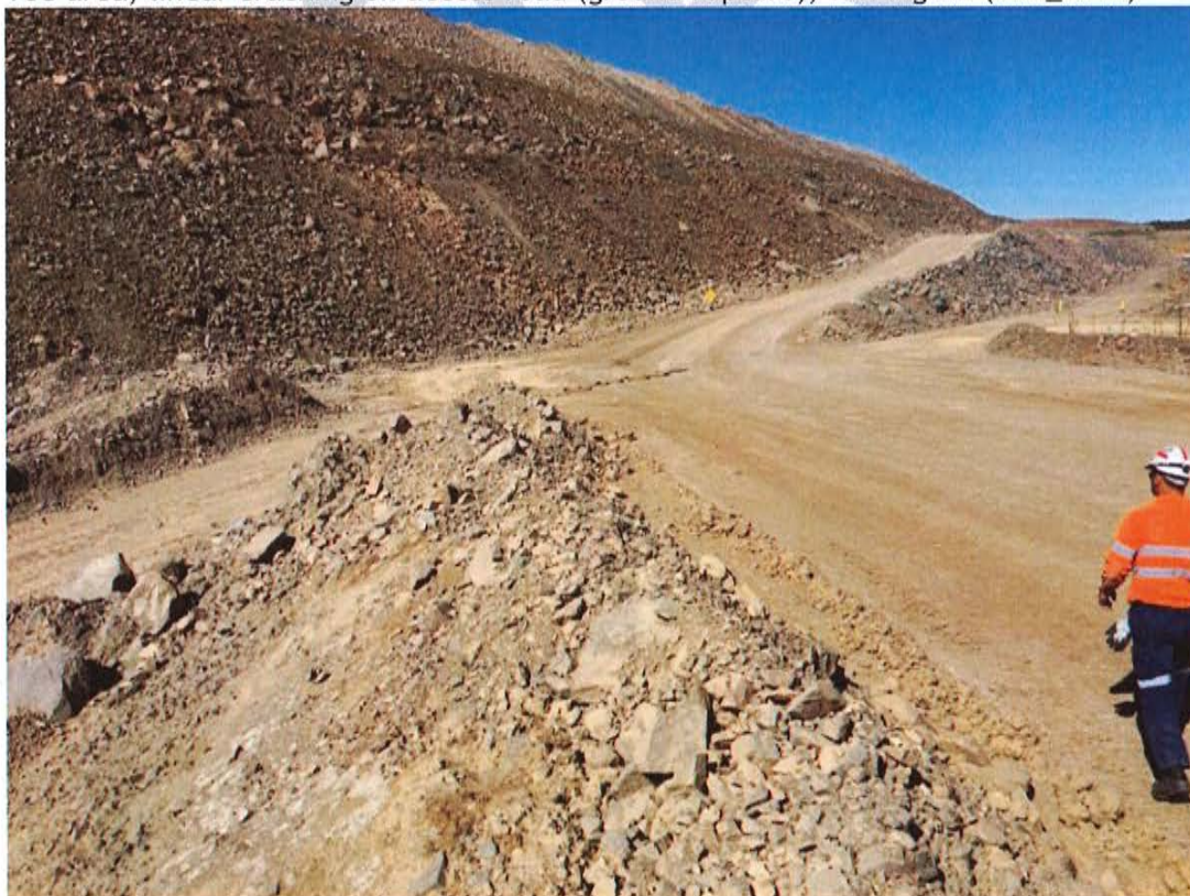
Toe area, linear cracking on access road (ground rupture), looking NE (IMG_2540)
