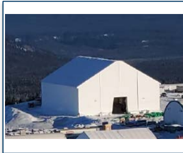
Improved working conditions for Red Chris employees with temporary workshop & long term warehouse
