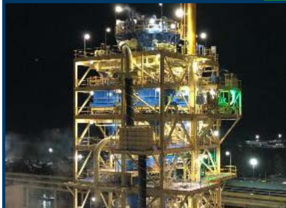
Float residue scavenging
